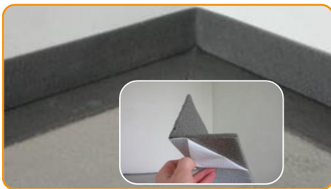
Insulate the concave corners with the "Profile" strip by cutting it as shown in the drawing.
