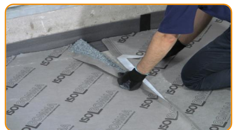
Seal the roll jointing borders by the adhesive flap available on the roll border. To do it properly follow the dotted and continues lines indication.
