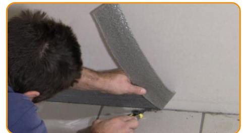
When the flooring application is completed, cut the exceeding part of the edging strips.
