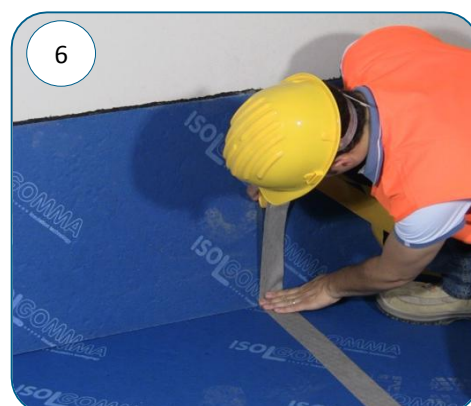
6 Seal the vertical joints of the mats with the Stik WP tape
