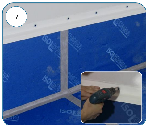
7 Fix the "Z" profile on the top border of the vertical mat
