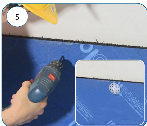
5 Fix the vertical mats with large headed screws or with adequate glue
