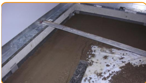
Melt the screed
