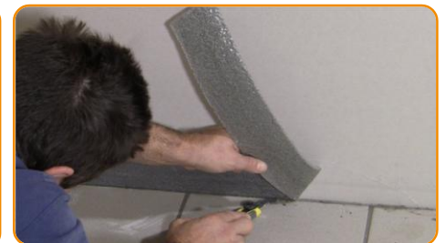
When the flooring application is completed, cut the exceeding part of the edging strips.
