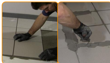
Lay down the final floor covering (ceramic or wood).
