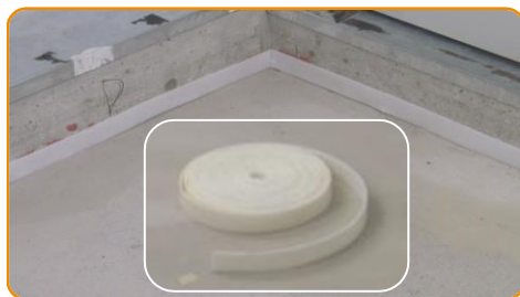
Apply the Profile Flat 5 all along the room perimeter.
